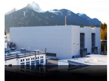
Construction of the Hot Rolling Mill Reutte Austria
